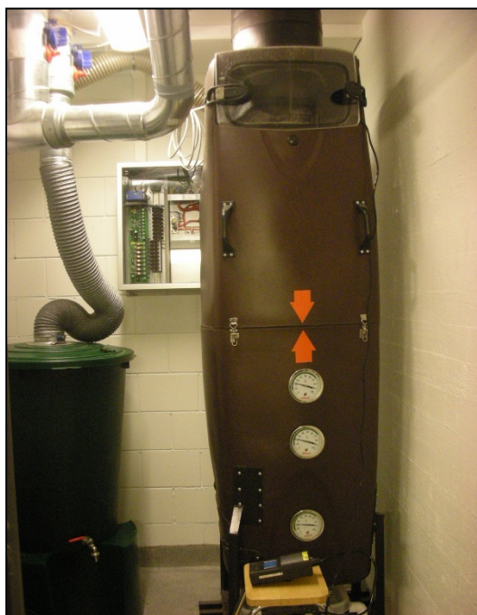
Picture 1. Dual-layer dry toilet composter
