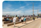
Arun East Bank flood defences, Littlehampton Environment Agency, Arun District Council & LDA Design
